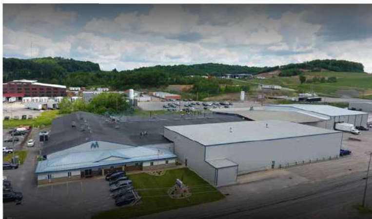
Fig. 1 Metco Industries' manufacturing facility on Bruxelles Street in St. Marys, Pennsylvania, one of the world's largest centres for press and sinter Powder Metallurgy production (Courtesy Metco)
